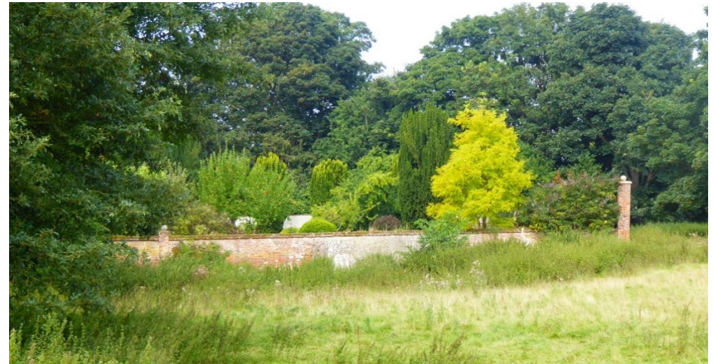
Figure 20: The garden wall at Chesfield Park
