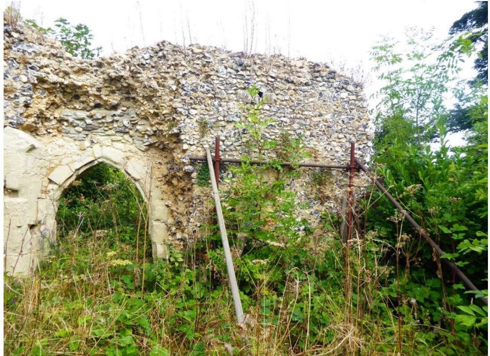
Figure 21: Scaffold shoring within the ruins of the Church of St Etheldreda
